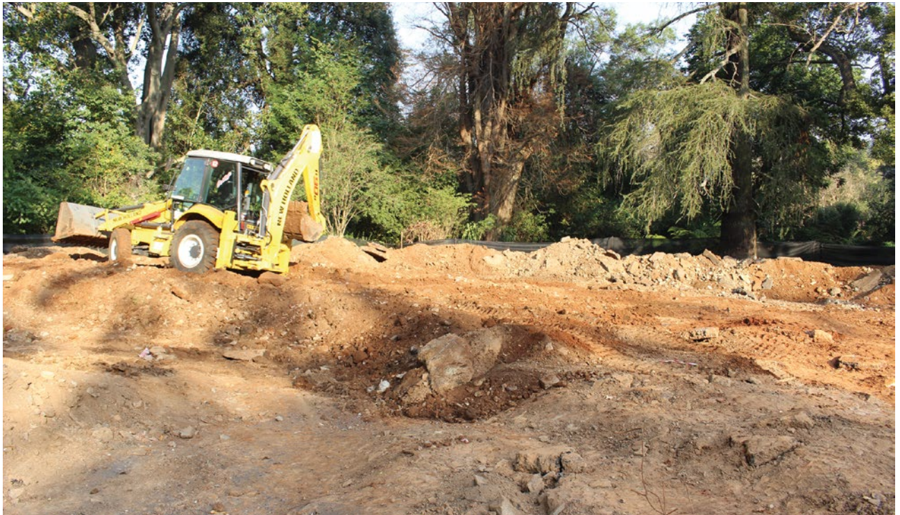
Figure 1. The new area to be converted into a home for the plants donated to the Pietermaritzburg Botanical Garden. Truckloads of soil were brought in and landscaped to turn the flat area into ridges with good drainage for cycads.
