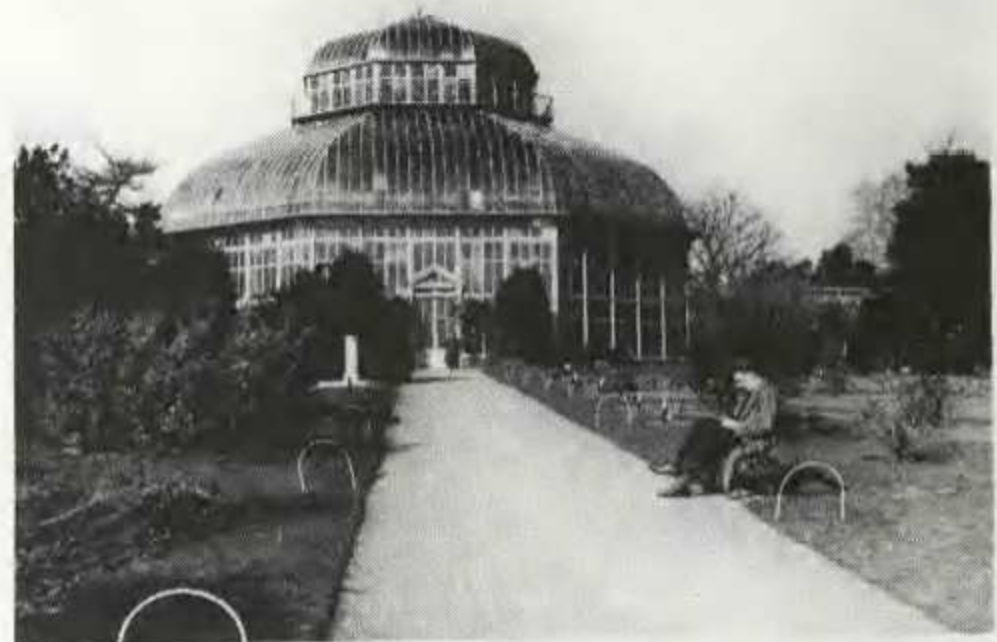
Figure 3 The Great Palm House (built 1884), National Botanic Gardens, Glasnevin, c. 1950.
