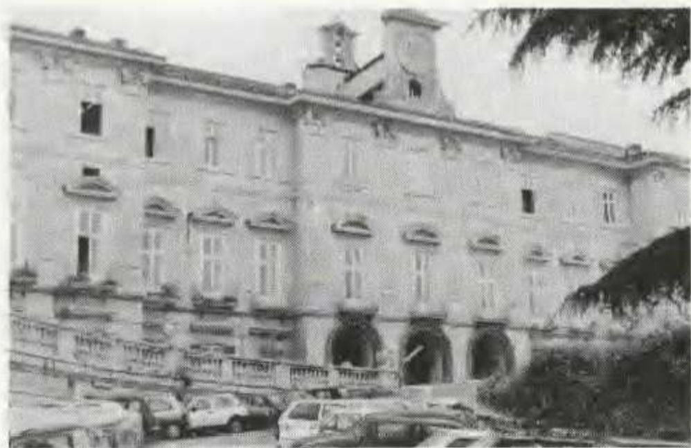
Figure 1 Part of the imposing Royal Palace of Portici. The botanical garden is to the rear of the Palace buildings.
