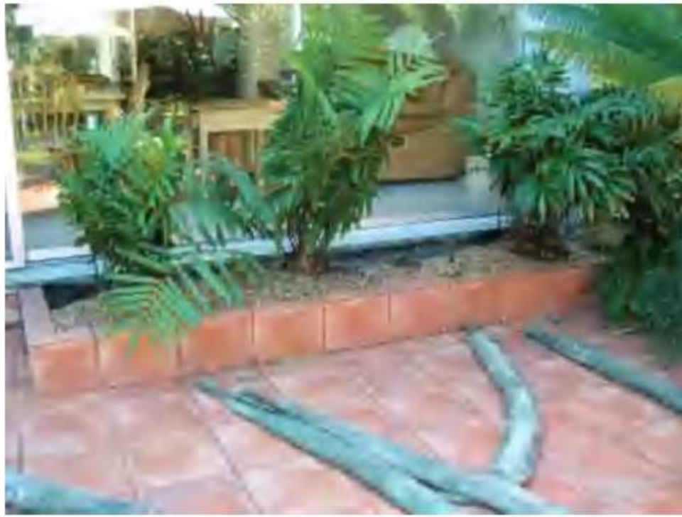
Figure 2.—: To allow the tarp to form a tight seal with the ground gravel, mulch or loose debris need to be swept away; note the sand snakes in the foreground that will be used to hold down the tarp edges.
